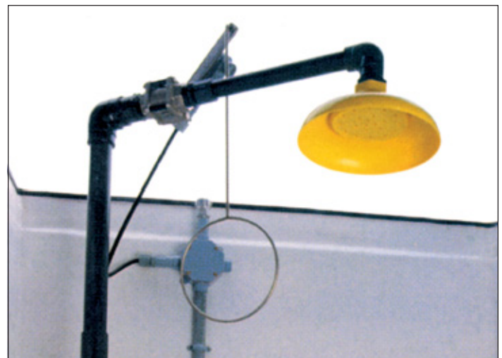
By pulling on the large ring, the shower delivers 113.6 litres/minute (30.0 U.S. gallons/minute, minimum 30 psi) of tempered water for a minimum of 15 minutes.
