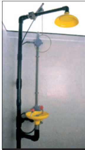
Shower/eyewash major components are constructed of corrosion resistant ABS plastic, stainless steel or chrome plated brass.
